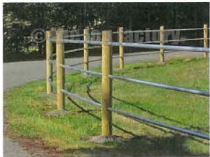
Typical timber post and galvanised steel rail horse fence www.thefactory.com.au
