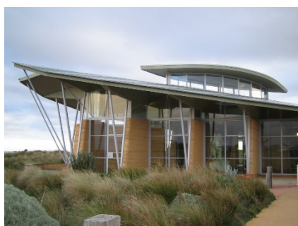
Openable roof top windows improve natural ventilation
