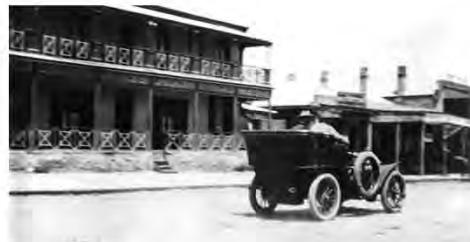
Albion Hotel in Wallace Street, circa 1910 - Note the original balustrading and footpath
