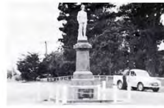
A View A-Looking east along Wilson Street Note:- white fence and footpath
