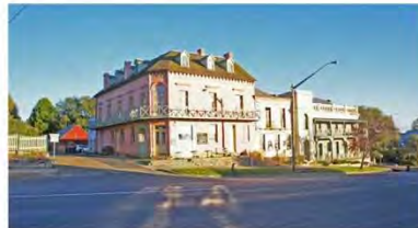
Note:- - changes to signage and awnings on first floor - balustrade and ramps to the streetscape no longer exist
