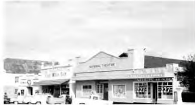
The National Theatre -Built as a roller skating rink circa 1936. - Photograph 1975.
