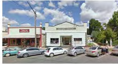
Note:- - the original awning and an adjoining shop front have been demolished
