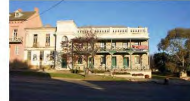
Note:- - changes to the verandah on building facade
