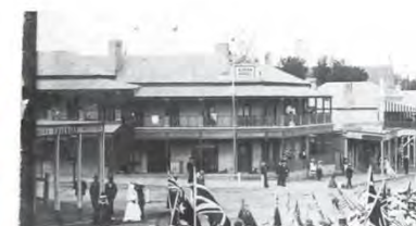
The Albion - built in 1872 as the 'Modern Hotel'
