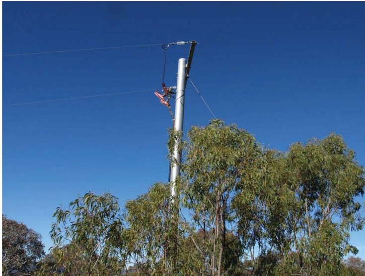
Figure 11. Golden wattles growing in close proximity to power lines near telecommunication tower.
