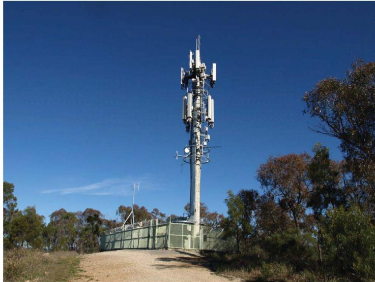
Figure 6. Location of telecommunication tower on Mt Jerrabomberra.
