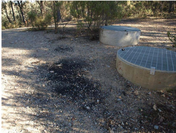
Figure 4. Evidence of a small fire at pumping infrastructure [E 701558 N 6083109].
