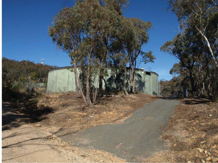
Figure 3. Location of Upper Thornton reservoir tanks on Mt Jerrabomberra.
