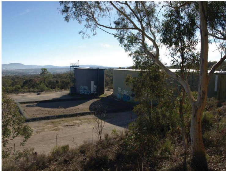
Figure 2. Location of water reservoir tanks on Mt Jerrabomberra.
