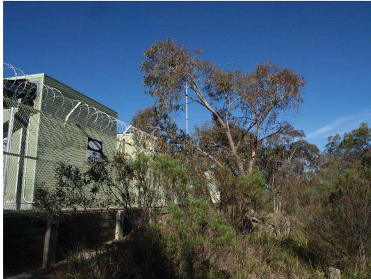
Figure 12. Vegetation encroaching into the telecommunication tower facility.
