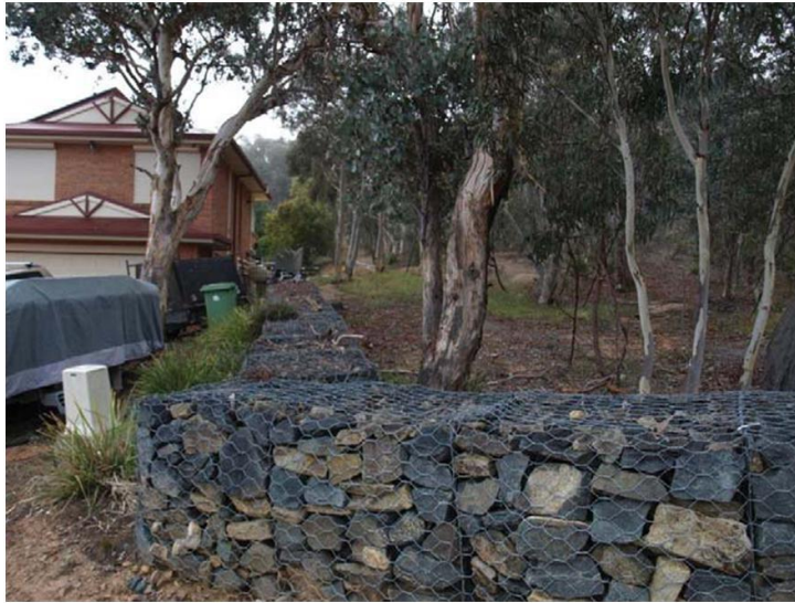
Figure 55. Properties with limited separation distance to bushfire hazard (APZ1).
