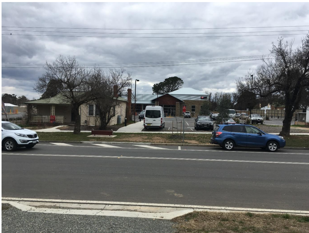
Figure 2: Adjacent Development (34 Malbon Street, Bungendore)
