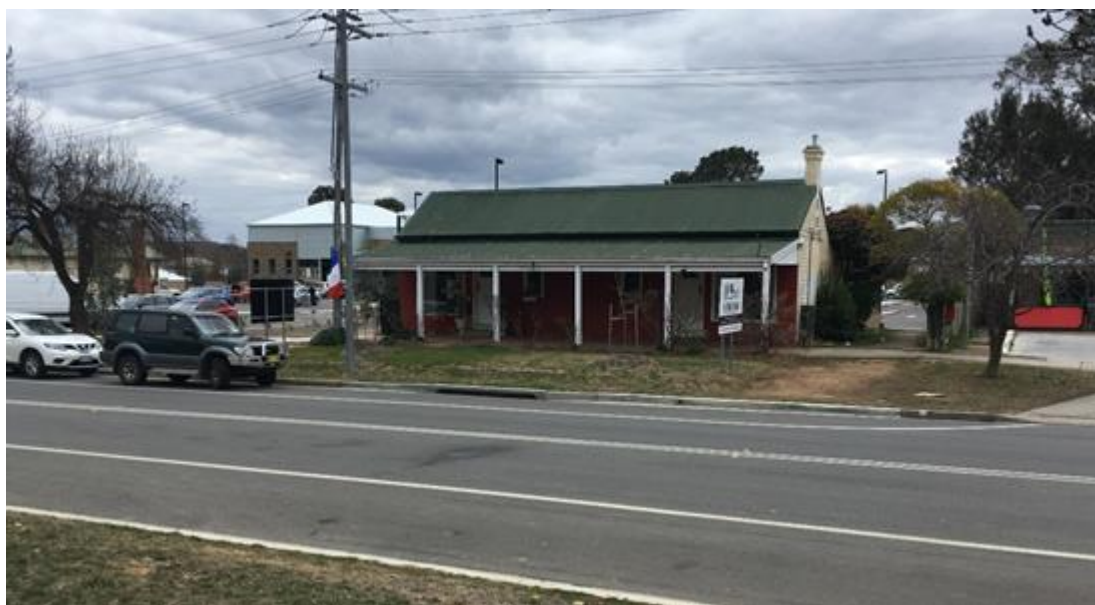
Figure 1: Existing weatherboard cottage (40 Malbon Street, Bungendore)
