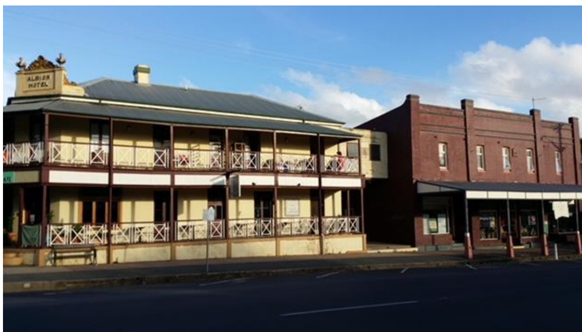
Figure 2 – Previous Configuration of Balustrades
