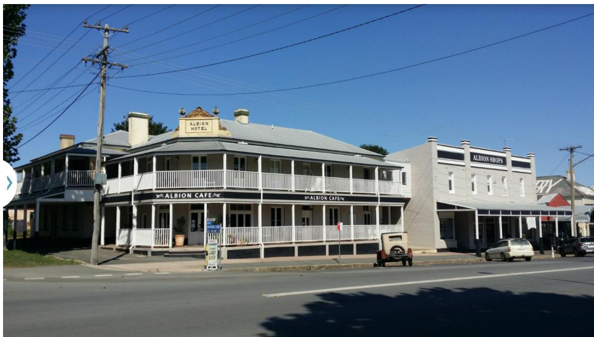
Figure1 – Present Configuration of Balustrades
