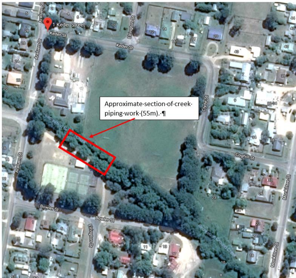
Figure 1: Aerial View of Braidwood Recreation Ground (Google maps) indicating the creek dissecting the site and approximate length of creek to be piped as part of this project.
