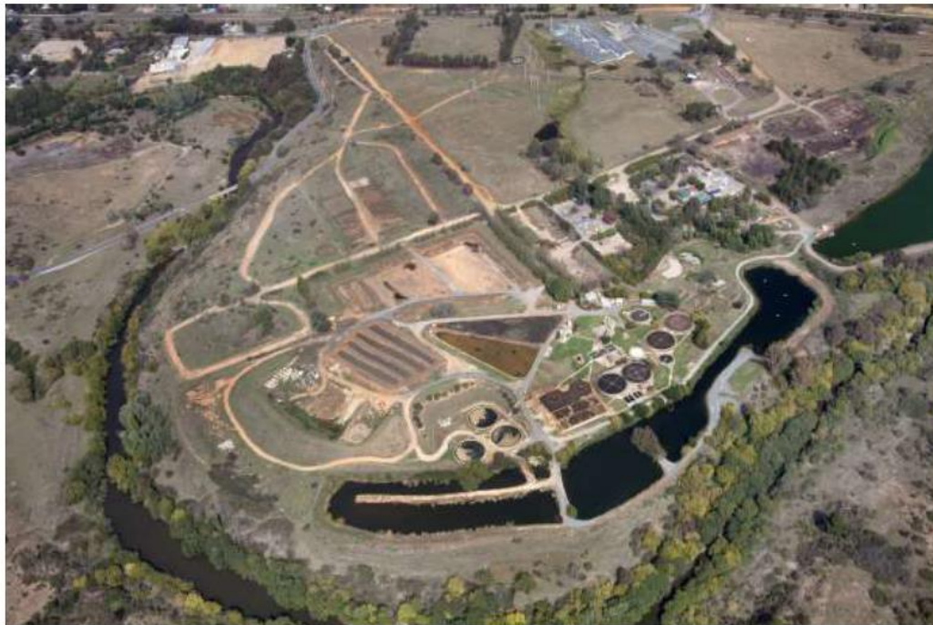
The current Queanbeyan Sewage Treatment Plant. Contracts were awarded for the concept design and project management services for the upgrade of the facility.
