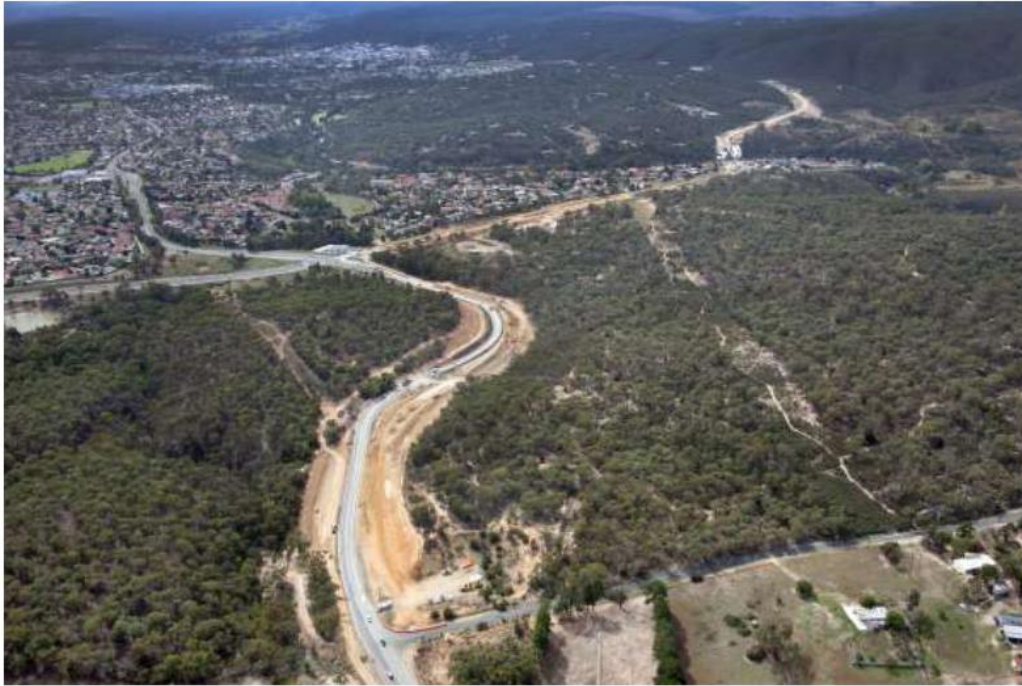
Construction of the Ellerton Drive extension in Queanbeyan made significant progress during 2018-19.
