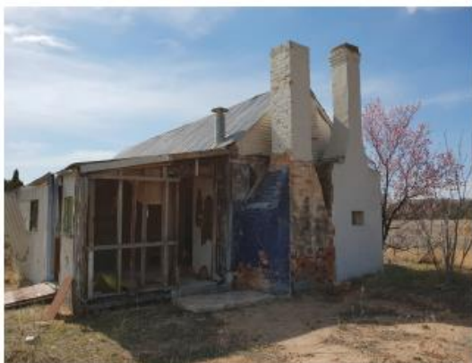
Existing Cook's Cottage Exterior
