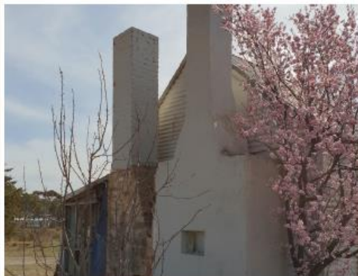
6. Existing Cook's Cottage Exterior
