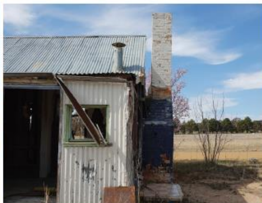
Existing Cook's Cottage Exterior)
