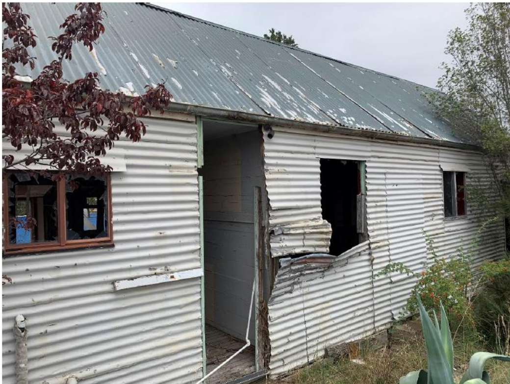
Figure 6 View of the Shearers' Quarters (Cook House) showing missing doors, windows and displaced wall fabric.
