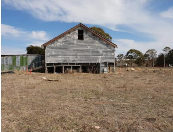
1. Existing Shearing Shed
