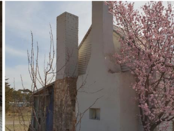
6. Existing Cook's Cottage Exterior
