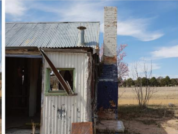
Existing Cook's Cottage Exterior)
