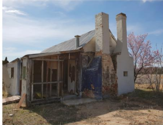
2. Existing Cooks's Cottage
