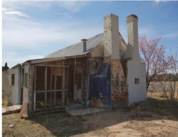
Existing Cook's Cottage Exterior
