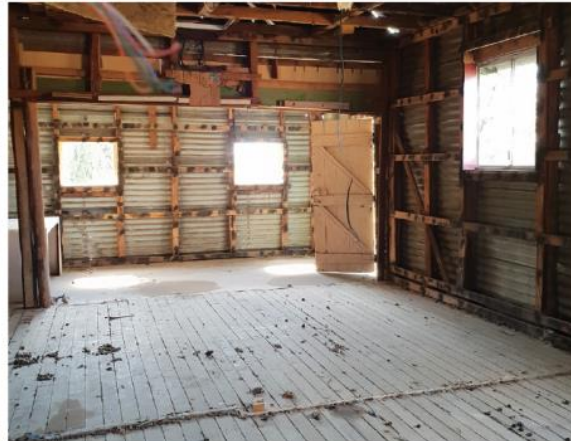
5. Existing Cooks's Cottage (interior)
