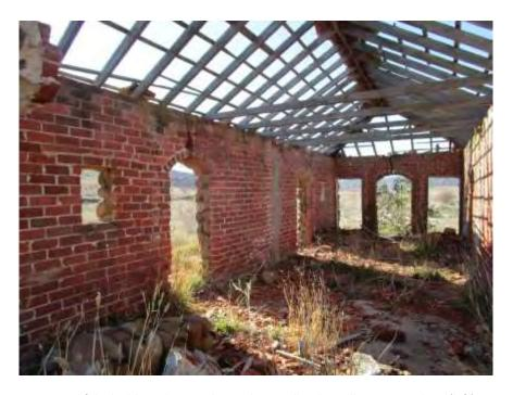
Interior of the building, showing the northern wall with small square windows (left), three entrances at the eastern end and the timber frame of the roof almost completely stripped of tiles
