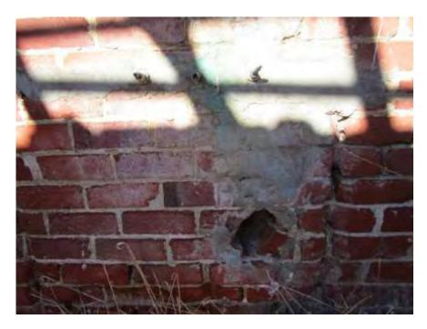
Metal pipes probably for taps protruding from the interior of the southern wall, with a large hole below into which a drainage pipe may have been fitted
