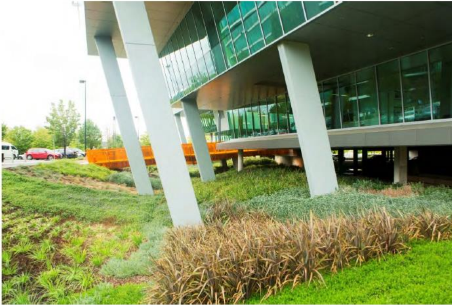
Figure 3.2- Landscaped swale, 3 Molonglo Drive, Brindabella Business Park
