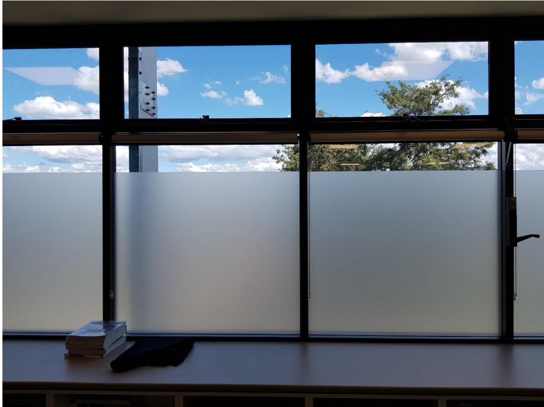
Figure 13: Detail of Obscure Glazing on Level 2
