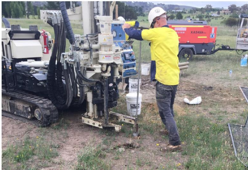
Figure 6 – Hand auger excavation in borehole MW02A. All boreholes were excavated/drilled using hand auger methods within the upper 0.5m bgl to minimise the likelihood of damage to underground services.
