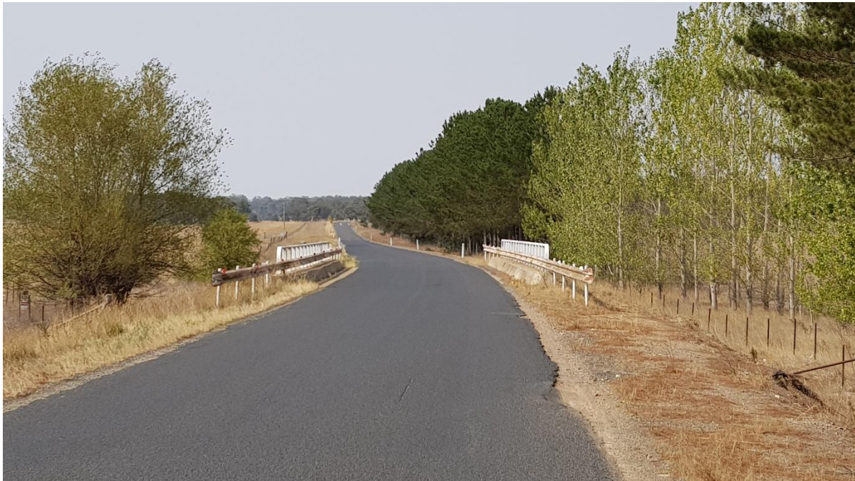
Figure 3 – Hoskinstown Road Bridge
