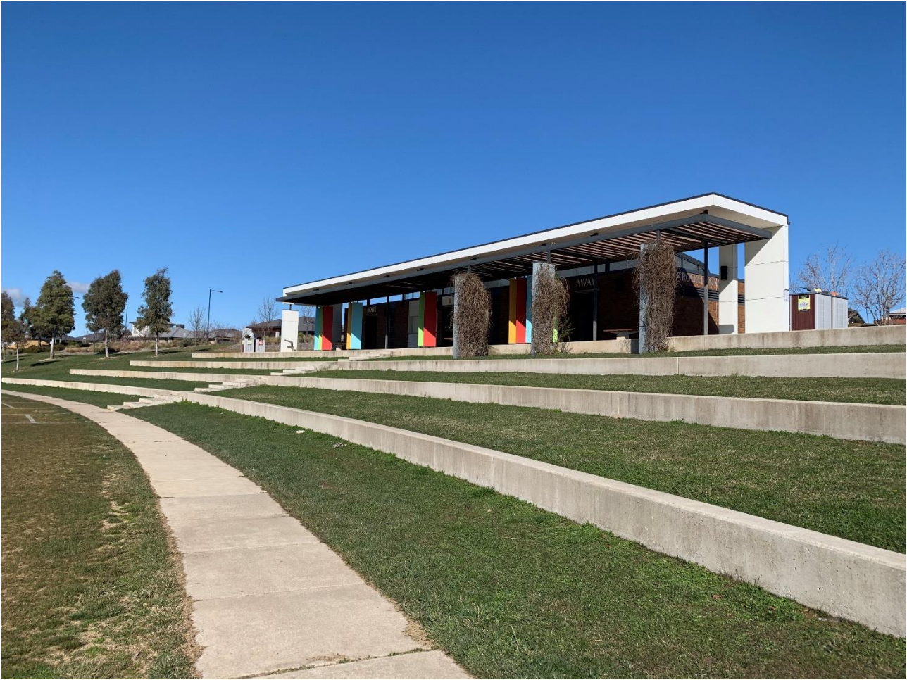
Figure 3 Rockley Oval facilities
