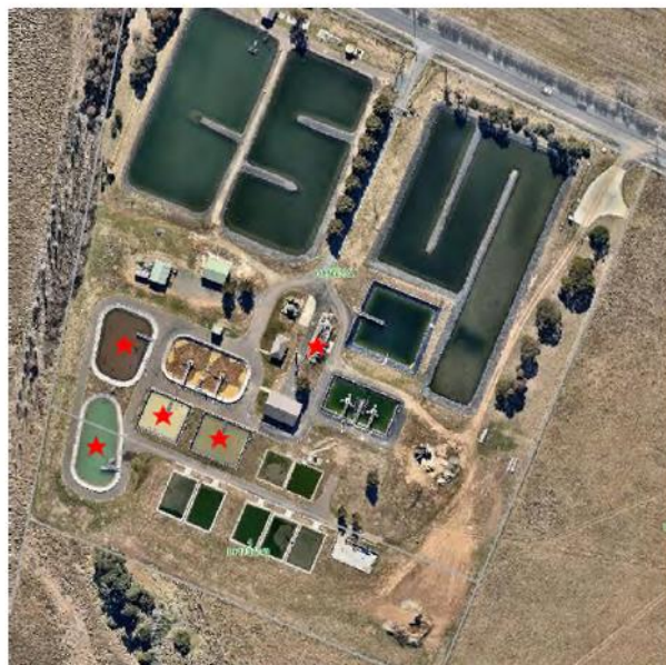
Bungendore Sewage Treatment Plant. Red stars indicating treatment processes which generate odour naturally, noting predominant west and north-westerly wind directions in Bungendore.
