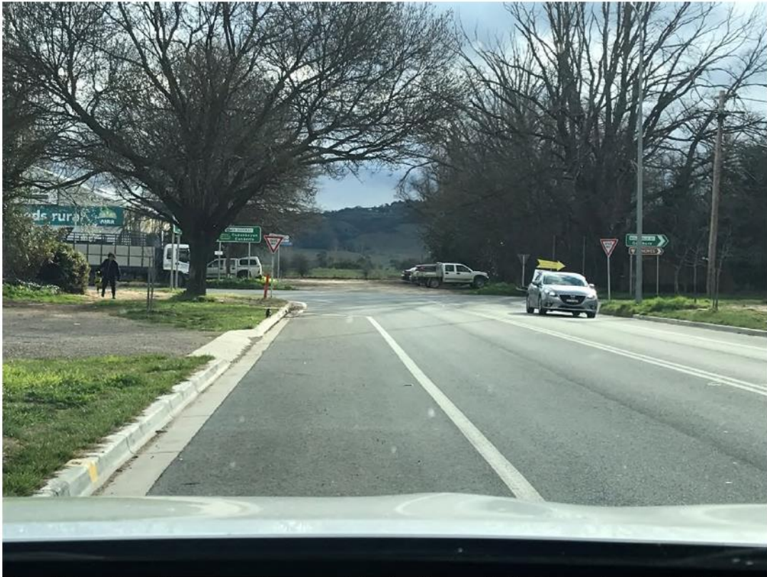
Figure 5: Location of the proposed new roundabout and access to the Bungendore Sports Hub.
