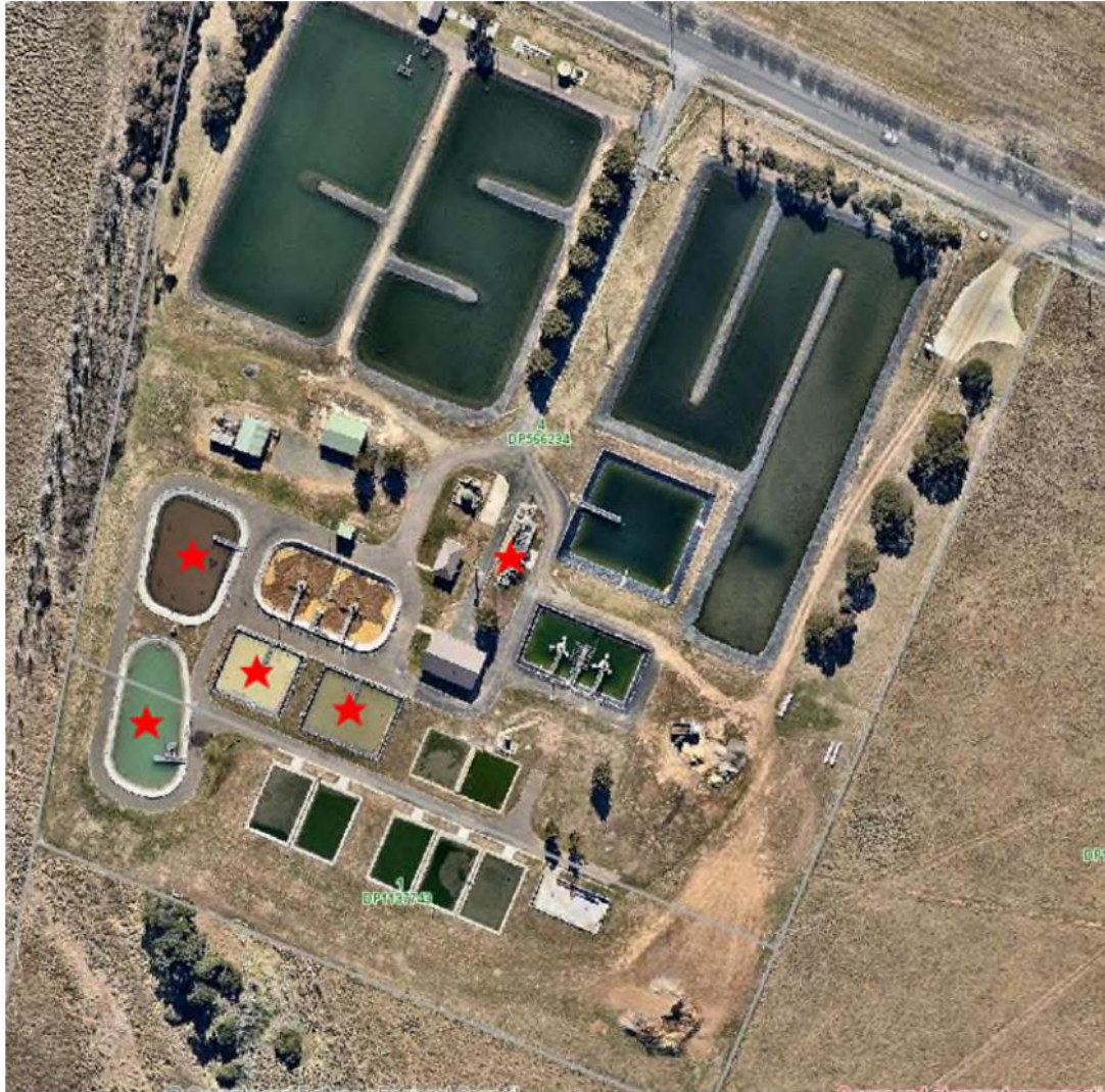
Figure 3: Bungendore Sewage Treatment Plant. Red stars indicating treatment processes which generate odour naturally, noting predominant south-westerly wind directions in Bungendore.
