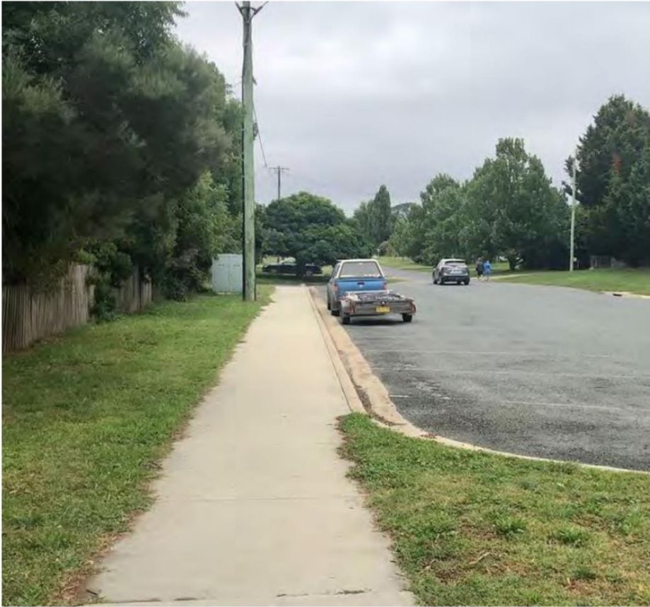
Despite a number of requests to unblock the drain in front of my house, nothing has been done. This is the result.
