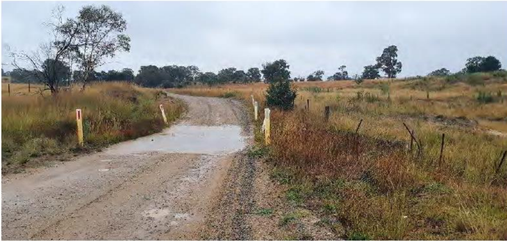
Culvert 1 – from East side
