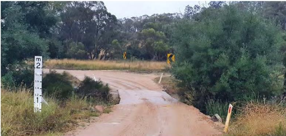
Culvert 2 – from south side
