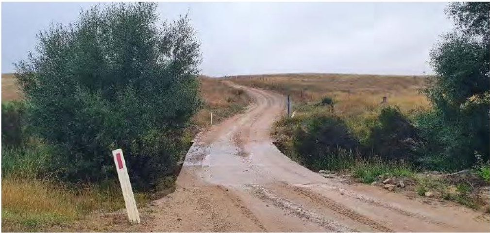
Culvert 2 – from north side
