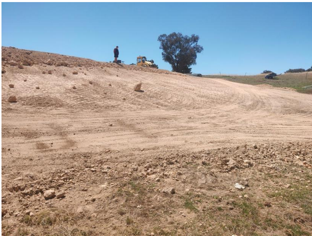
Figure 3: Fill Used to Level the Proposed Siting of The Farm Building
