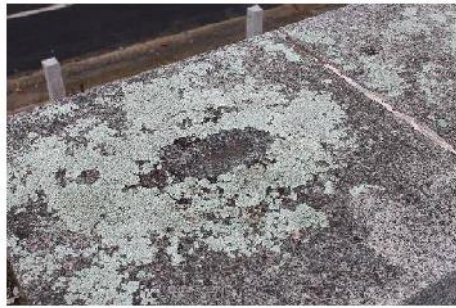
Lichen growth at top of memorial around an indent in the stone surface
