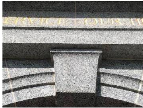
Surfaces cleaned and joints regouted
