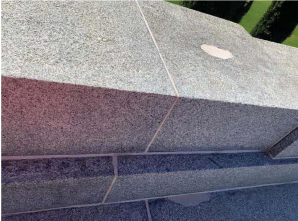
SHOWING PATCHING OF SPALLS AND CLOSEUP OF JOINTS USING WESTOX REPOINT.
