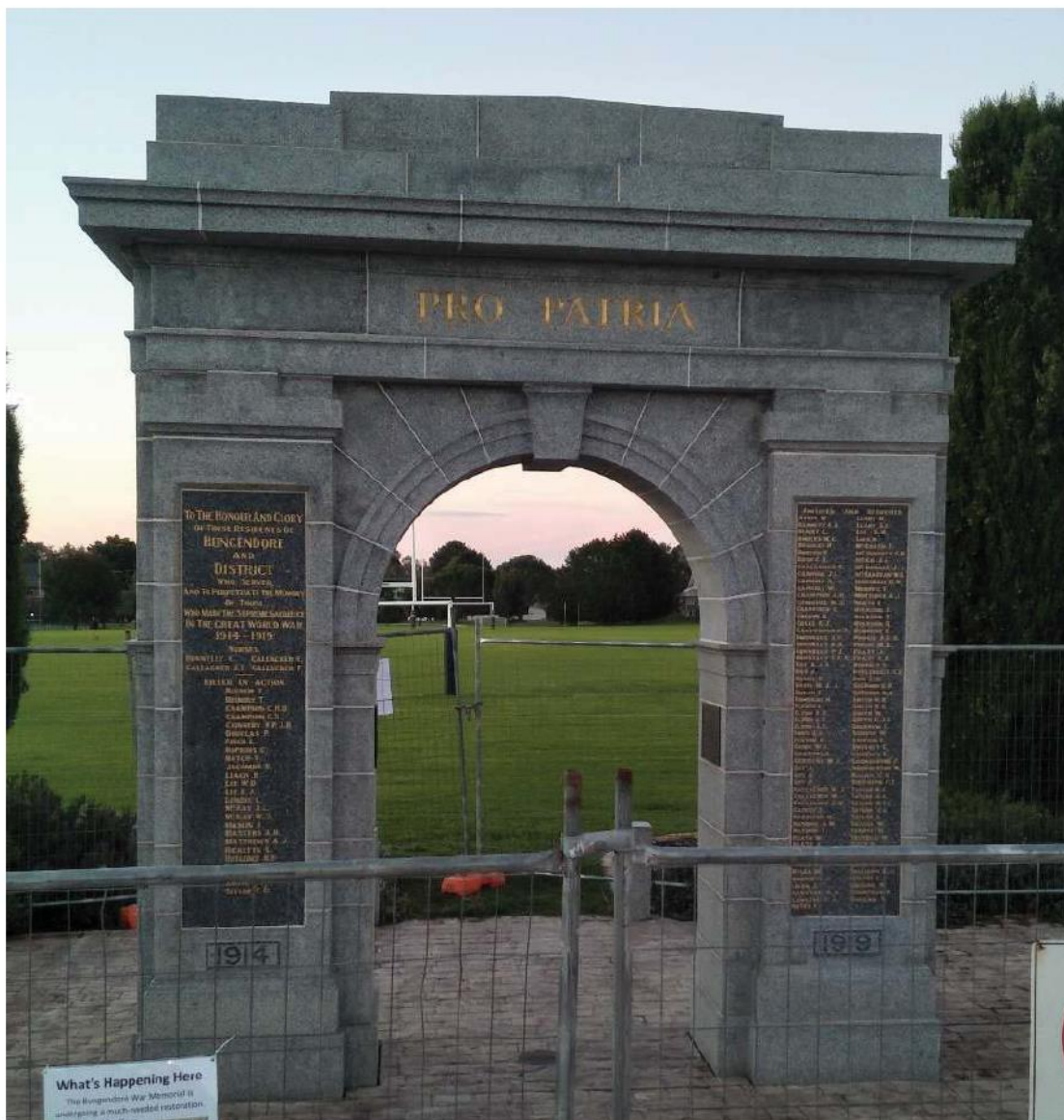
COMPLETED RESTORATION – SOUTH ELEVATION.
