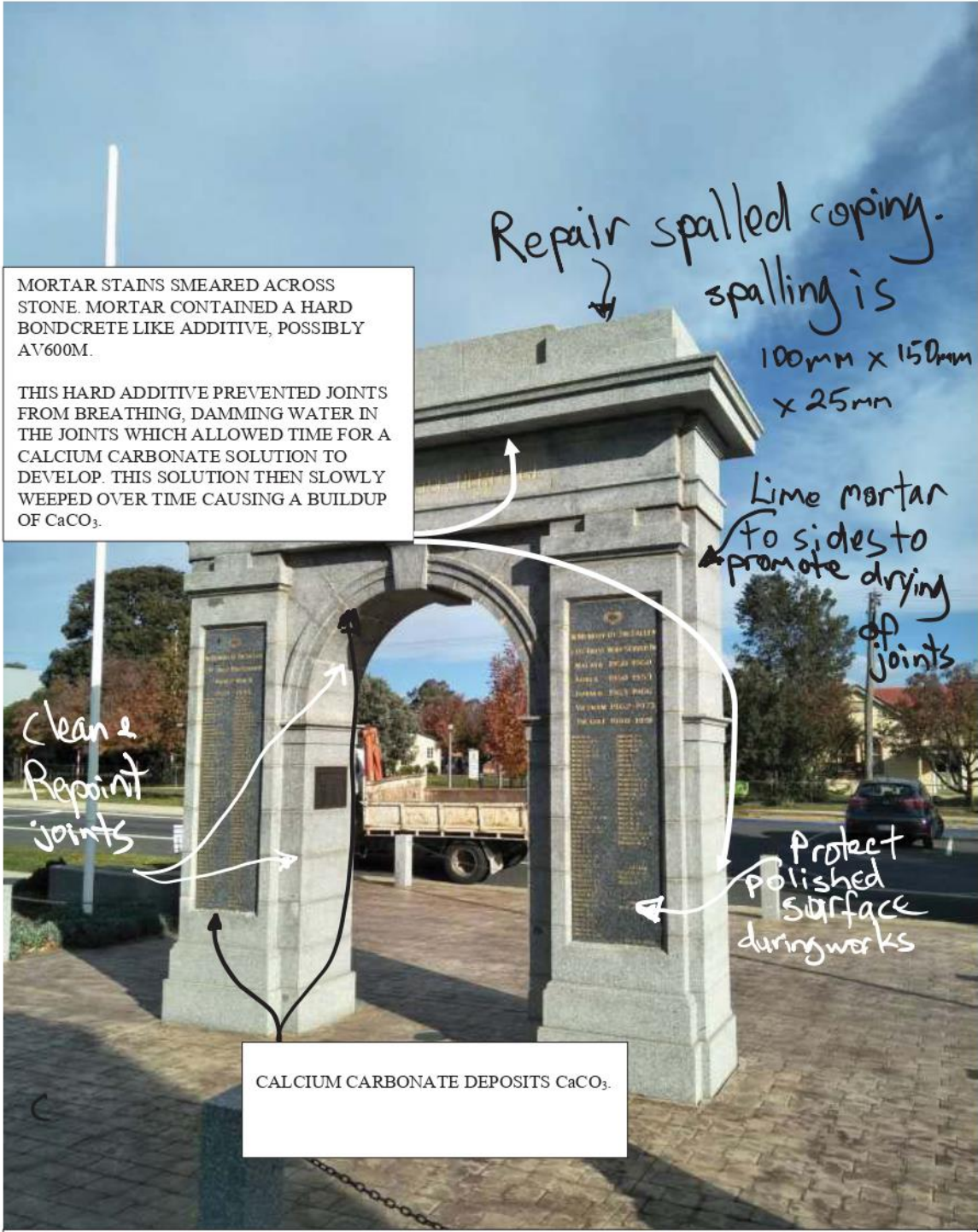
CONDITION PRIOR TO CLEANING – NORTH ELEVATION
