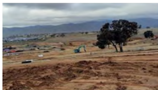
Poor erosion/sediment controls on subdivision site.
