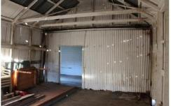
Western shed showing connection into the eastern shed. The wall and gutter of the eastern shed is visible, suggesting it was built first.
