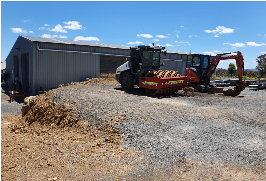
Figure 2: Site View (North West) 16 Nov 2021
