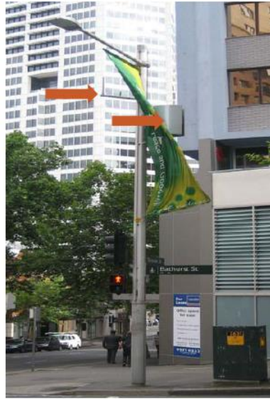
A microcell omnidirectional antenna attached to an existing street light pole (extending to the left under the light) and accompanying equipment unit (attached to the right).
