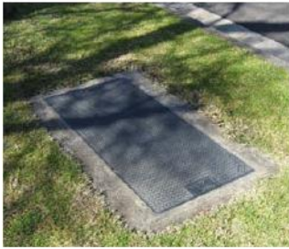
Example of underground housing for telecommunications facilities.
