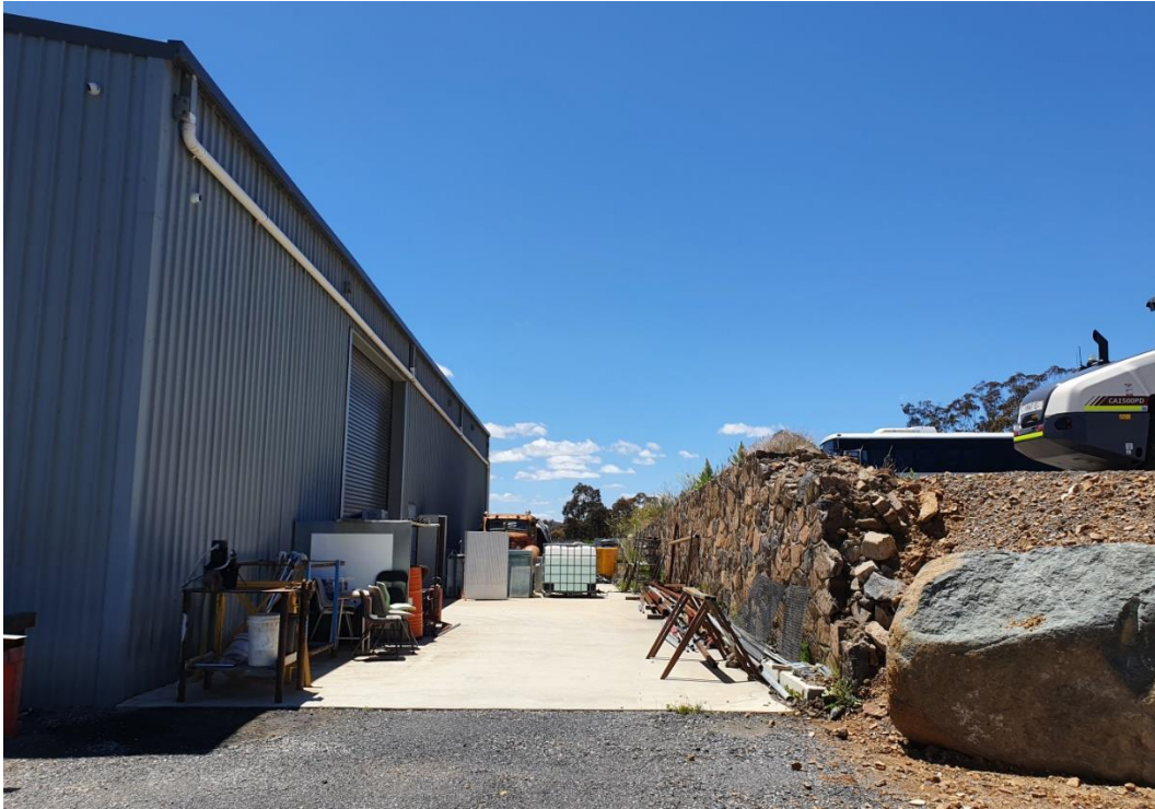
Figure 5: Site View (North East) 16 Nov 2021
