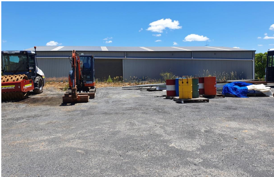
Figure 4: Site View (South) 16 Nov 2021
