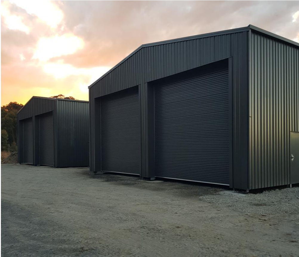
Figure 6: Proposed sheds built on site without DA determination (photos sent to council by applicant on 08 Feb 2022)
