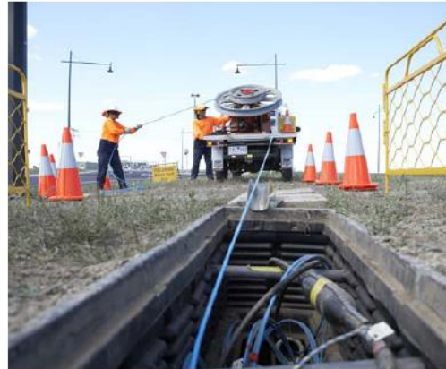
Cable being inserted into duct.
