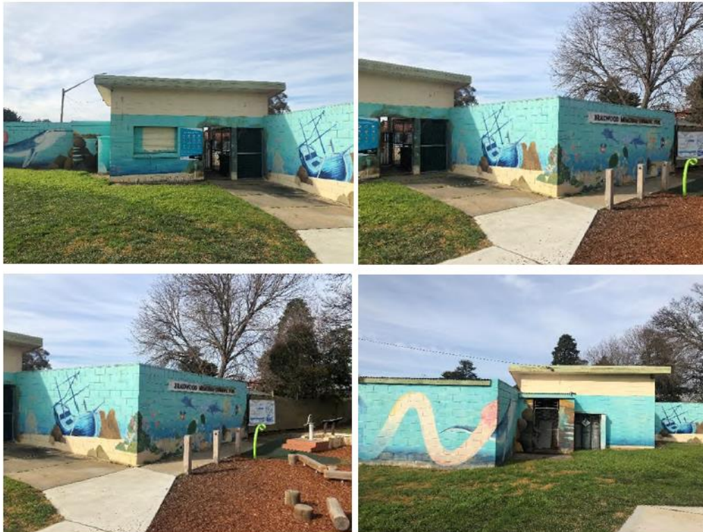
Figures 2-5: Site photos of existing swimming pool and facilities
