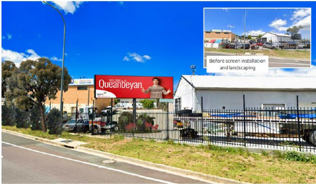
Figure 6: Photo shows proposed amended location of digital advertising sign which partially blocks advertising sign on adjoining building. Also depicts proposed landscaping on Council's road reserve.
