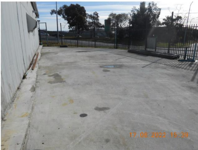
Photo shows concreted area in front of existing building that will be difficult to access.
