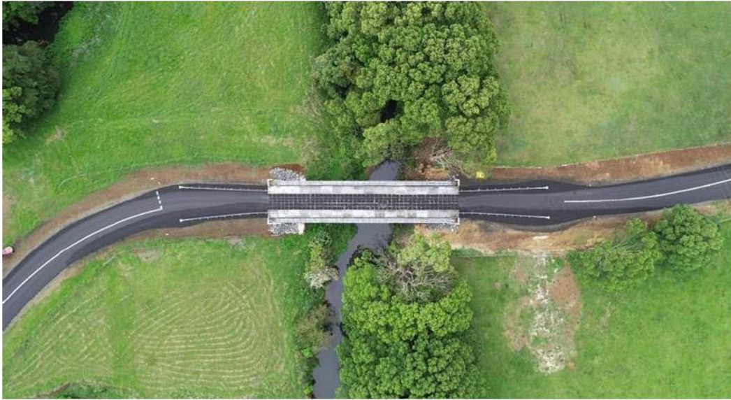
Brookers Bridge pre-upgrade, Singleton NSW
