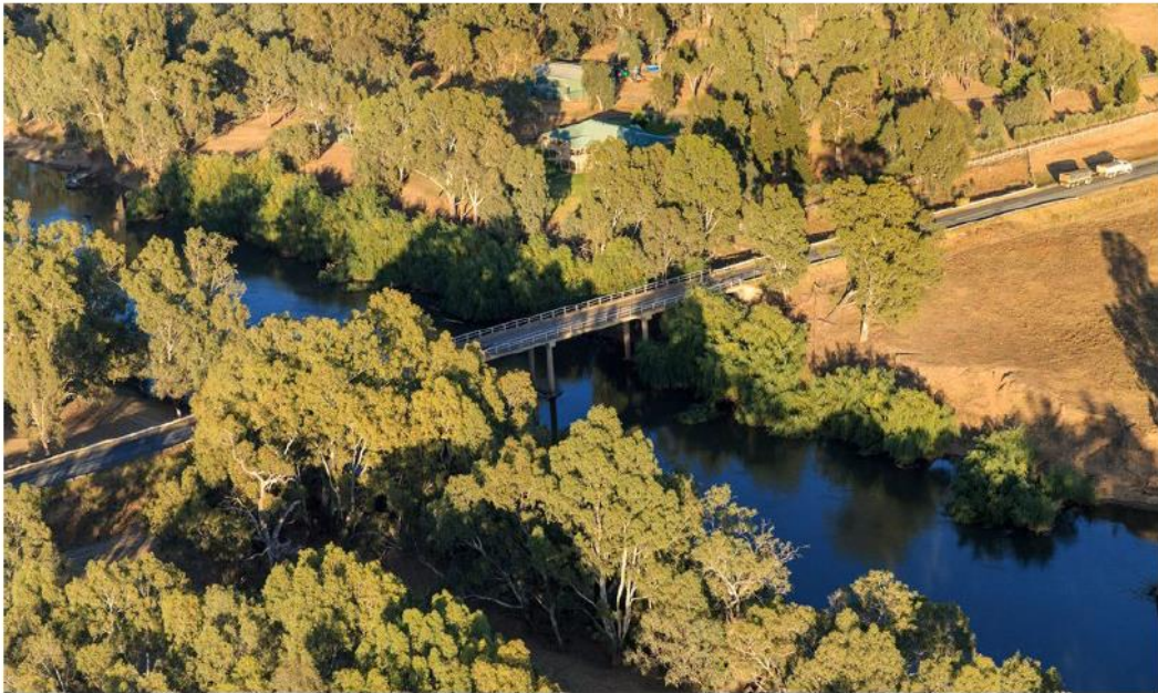
Tenterden Road Bridge, Guyra
