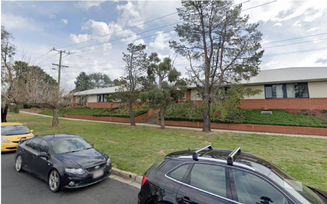
Figure 2: The Building's Entrance from Erin Street
