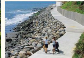
New Plymouth Coastal Walkway, 1999
