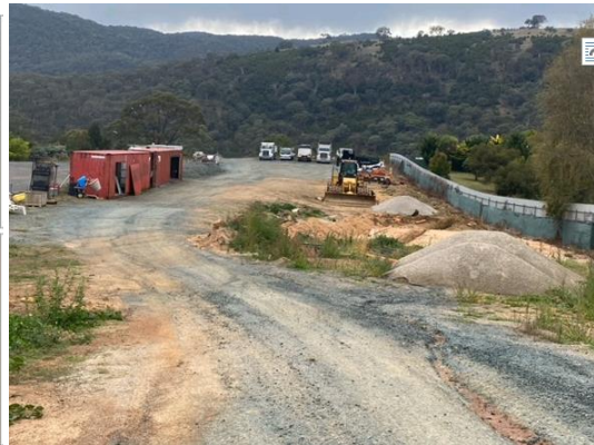
Shipping containers and trucks on site
