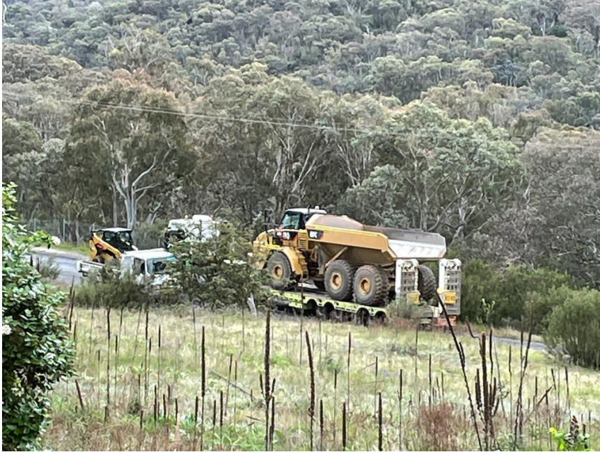
Figure 3 – BASE Construction Pty Ltd plant being transported along Wickerslack Lane
