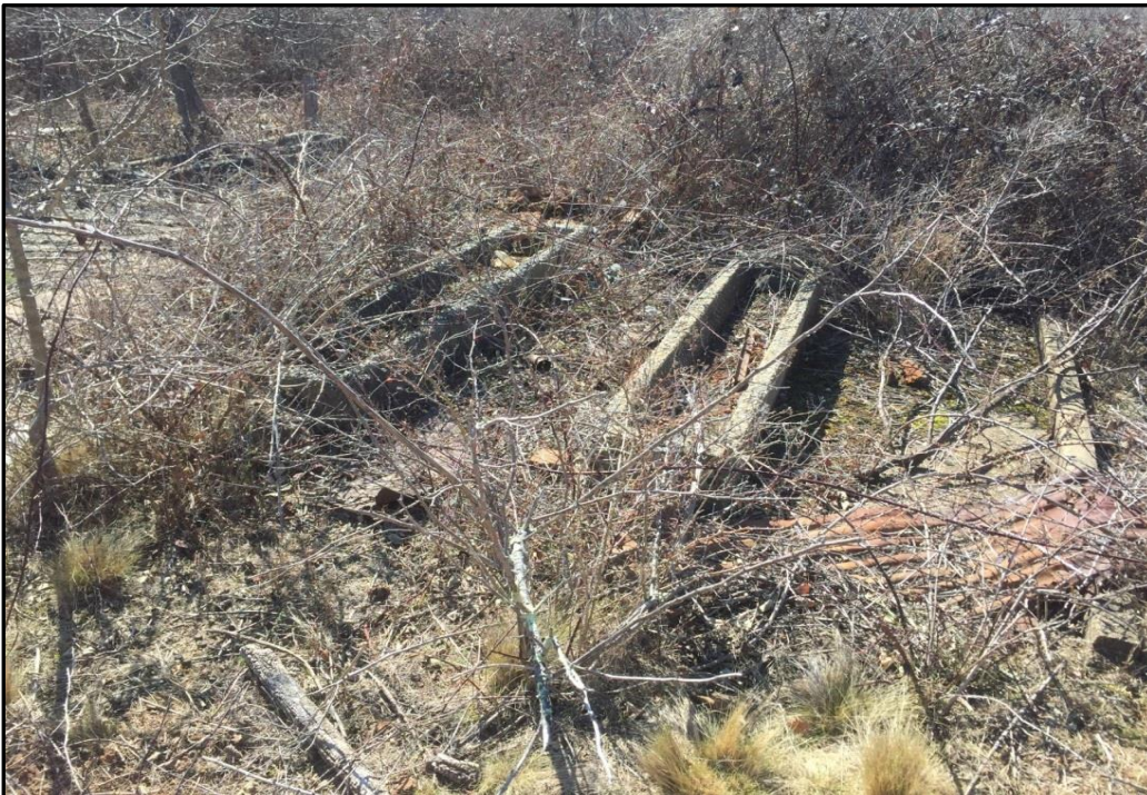
Photo 24: View of Mineral Processing area, example of concrete troughs
