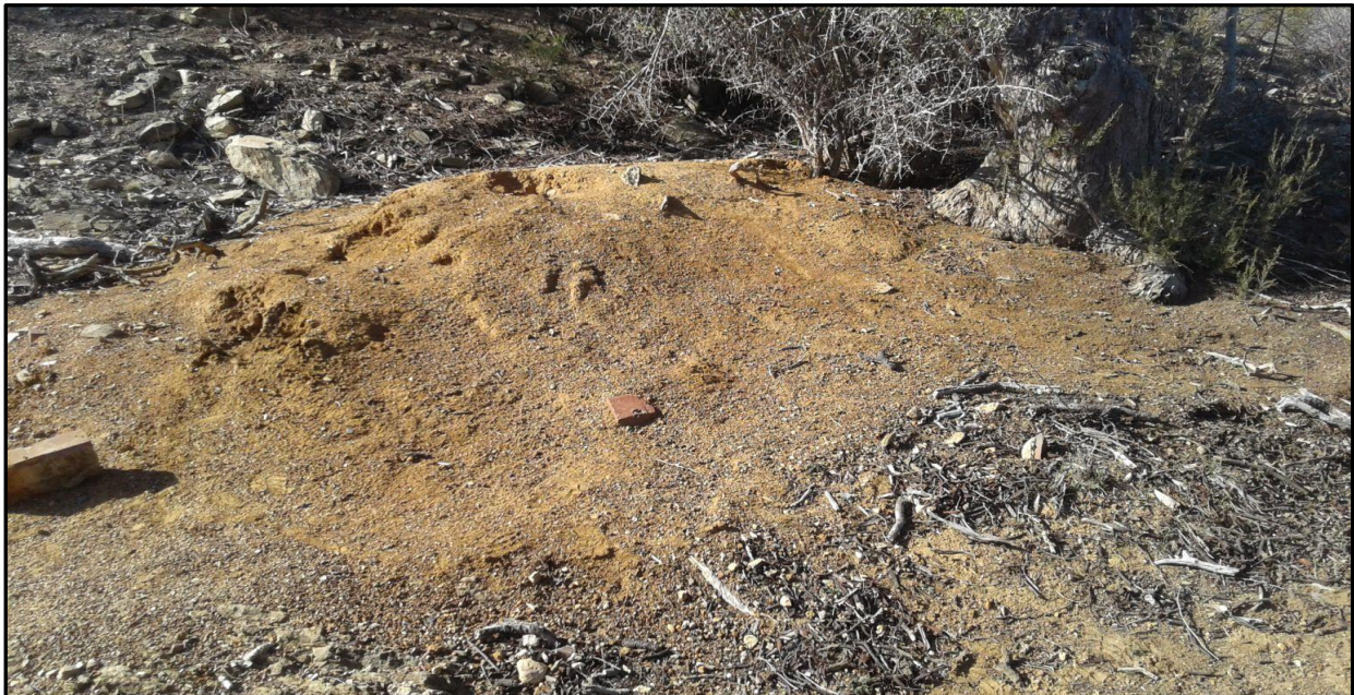
Photo 36: View of small stockpile in east of the site containing asbestos material
