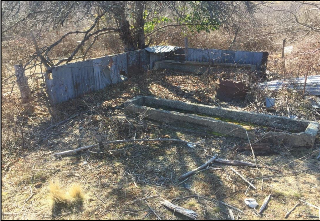
Photo 25: View of Mineral Processing area, remnant buildings
