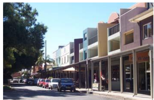
Shop top housing Sawtell NSW
