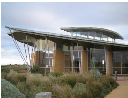
Openable roof top windows improve natural ventilation
