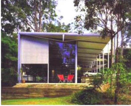
House with large windows facing north maximise solar access and verandah down the western façade to shade from summer afternoon sun.
