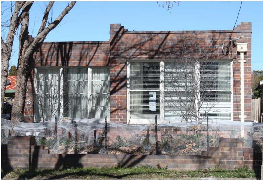
Figure 10: Inter-War Modernist style with flat roof, decorative parapets and large windows with horizontal glazing bars.
