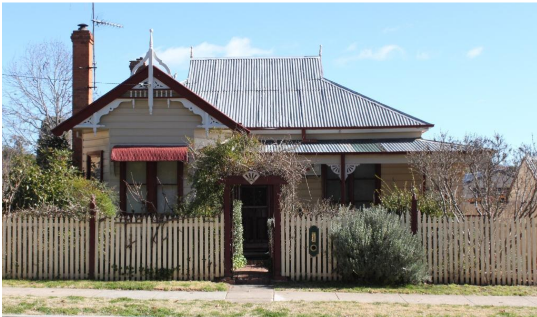
Figure 8: Federation style cottage with small gables in roof, finials and decorative barge boards
