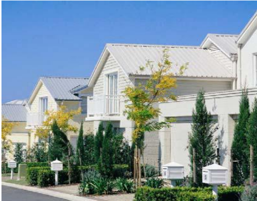
Garage set back to rear laneway
