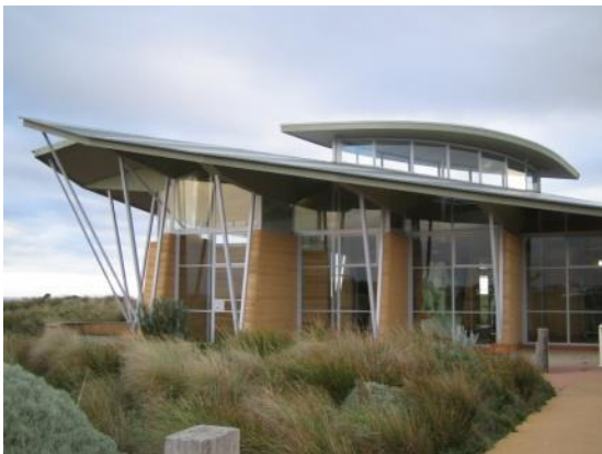
Openable roof top windows improve natural ventilation
