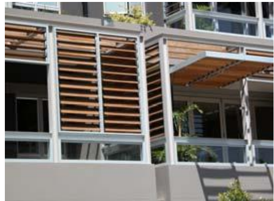
Dual purpose sun shading and ventilation external louvers
