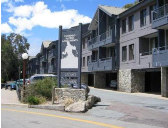
Basement Parking entries incorporated into design of residential flat building
