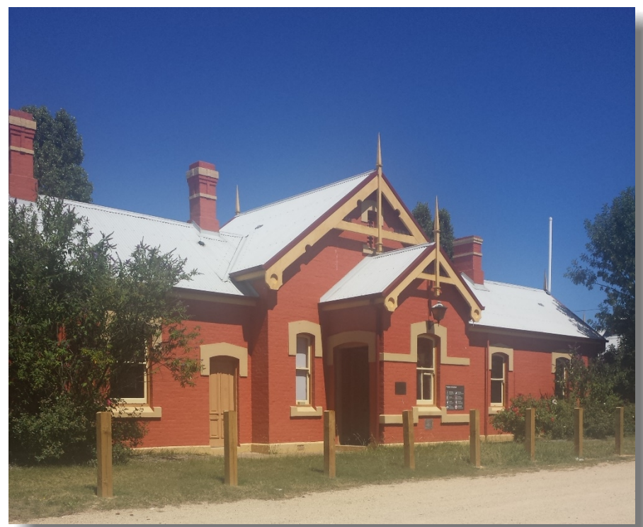
Photo 1 Bungendore Railway Station
