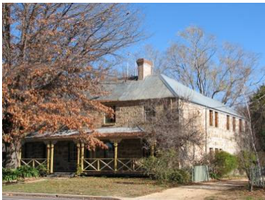
Old Stone House (Molonglo Street) – unique two storey painted stone house built by John Donohue in 1867.
