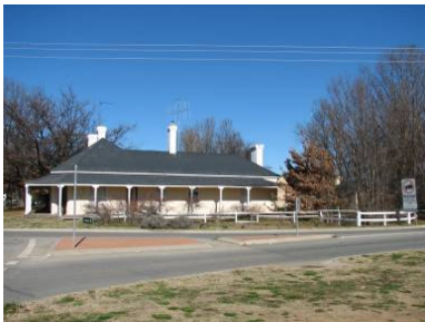
Old Commercial Bank (cnr Molonglo and Gibraltar Streets) – substantial single storey rendered stone building with corrugated iron roof, verandah along main street frontages and outbuildings, constructed 1850-90 period.
