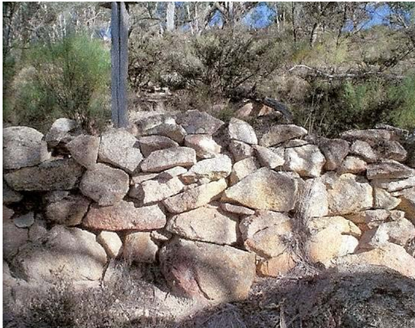
Burra Station Dry Stone Wall Burra Station Boundary Marker p14 2008
