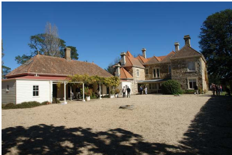
Rear façade - Currandooley Homestead
