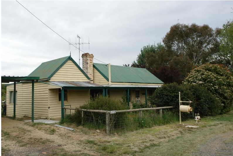
1712 Hoskinstown Road, Hoskinstown
