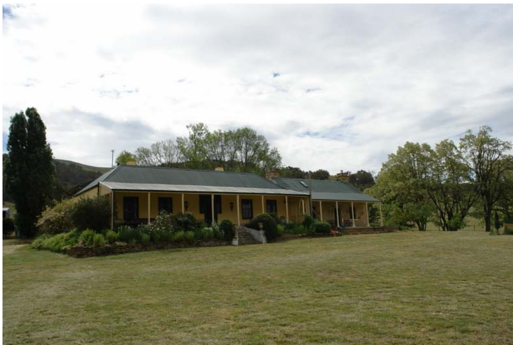
The Briars 1843 house at right
