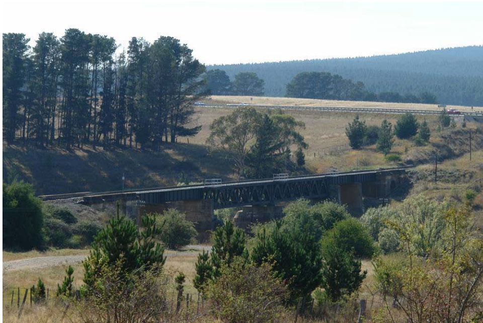
Burbong Railway Bridge over the Molonglo River
