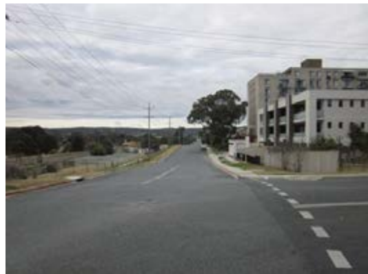
Figure 2.5: Henderson Road Looking East
