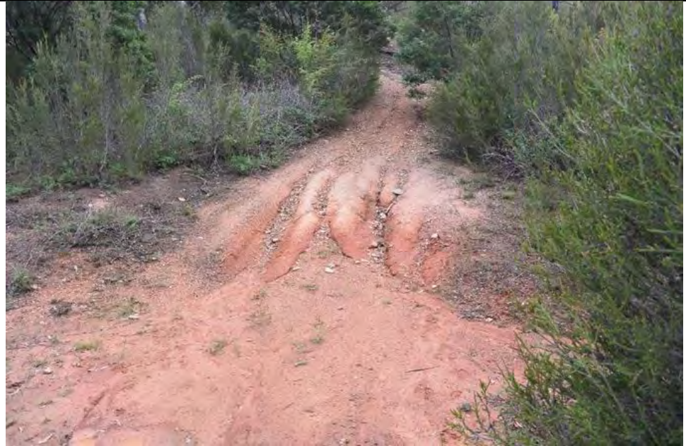
DSC 3770: Wheel rut erosion and deposition in channel of crossover
