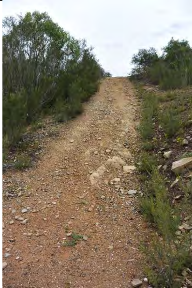
DSC 3768: Minor wheel rut erosion
