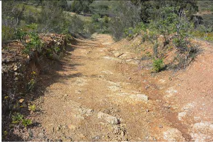
DSC 3799: Deeply incised trail concentrating run-off
