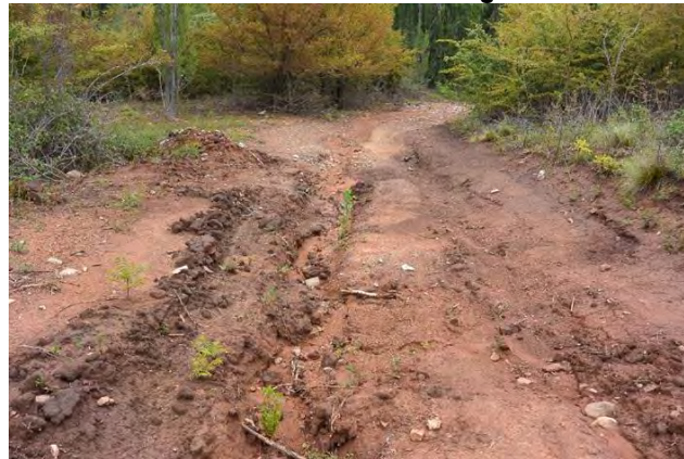
DSC 3781: Deeply rutted areas will require building up with topsoil
