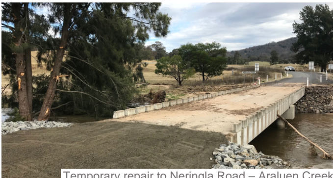
Temporary repair to Neringla Road – Araluen Creek
