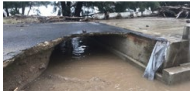
Flood damage on Neringla Road August 2020
