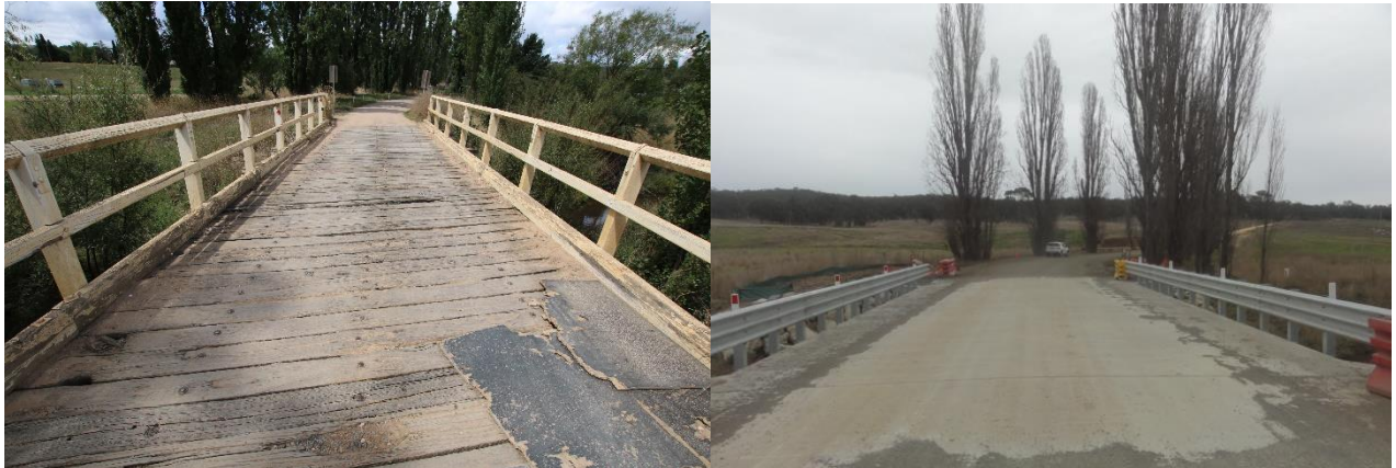
The former Gidleigh Bridge and the upgraded, concrete bridge which was completed in May 2021.
