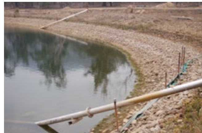
Braidwood off-river storage dam January 2020
