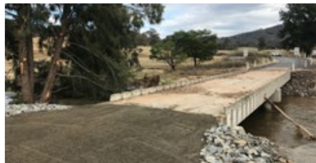
Temporary repair to restore access (Neringla Road) August 2020
