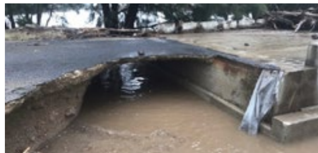
Flood damage on Neringla Road August 2020
