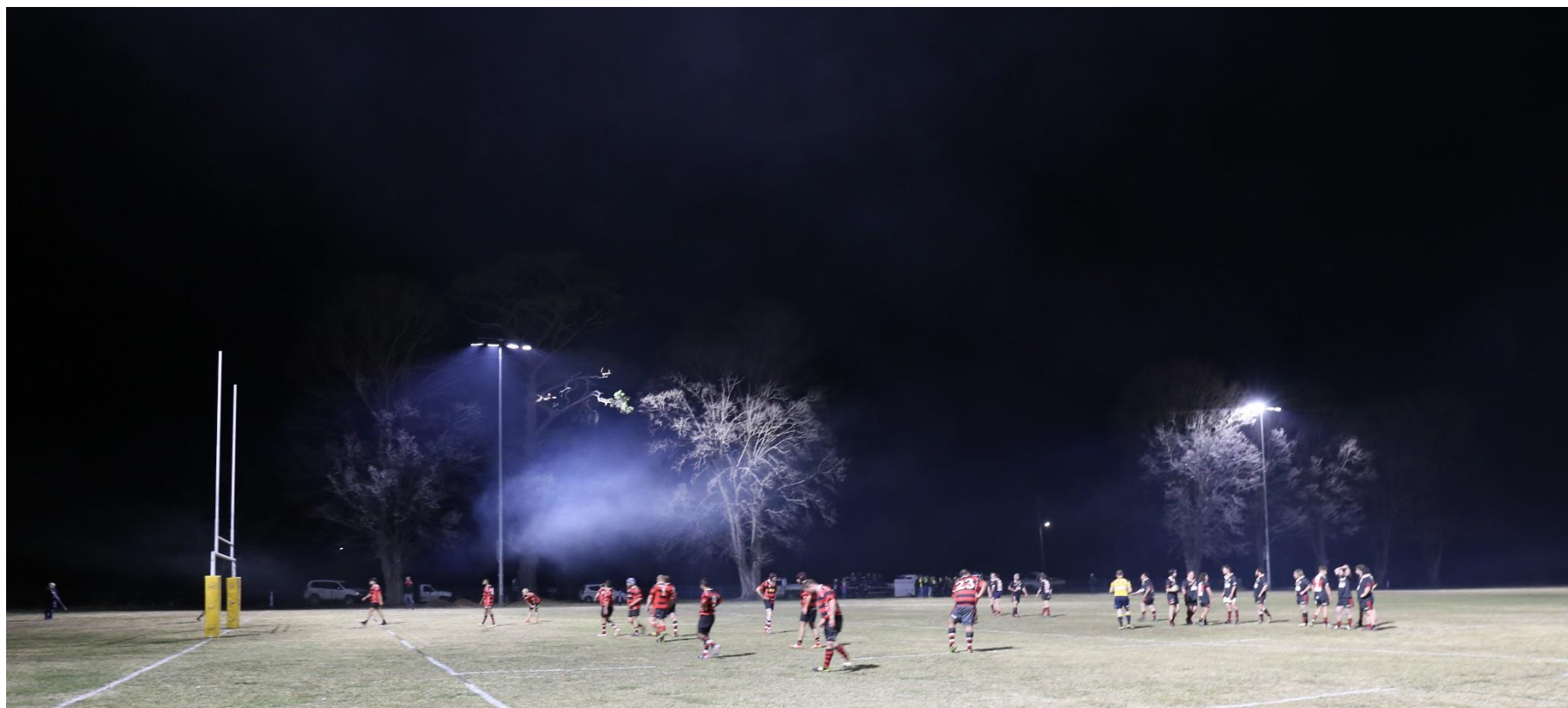
New floodlights were installed at the Braidwood Recreation Ground, with the first match played under lights in August 2018.
