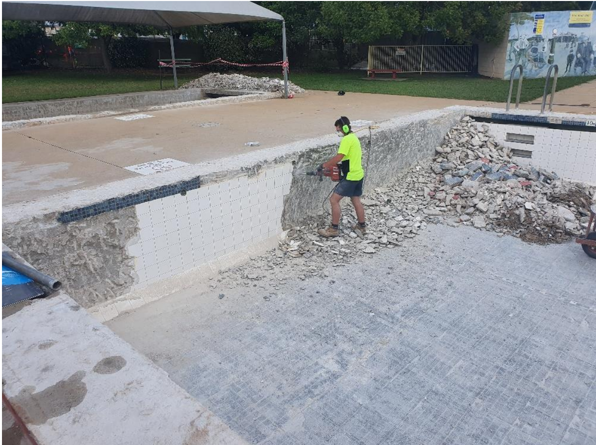
The tiles on the Braidwood Pool were replaced as part of the refurbishment project in mid-2020.
