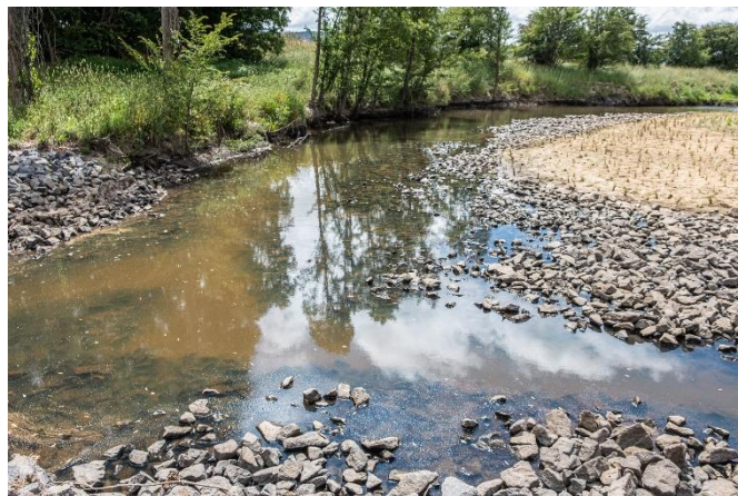
Works associated with the Bungendore Flood Risk Management Plan were undertaken at the intersection of Turallo and Halfway Creeks in Bungendore.
