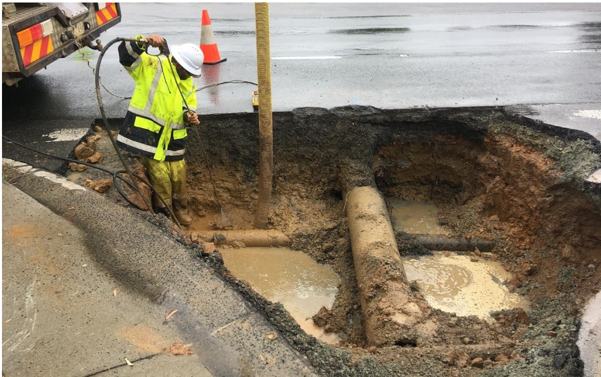
Staff work on a broken water main in Queanbeyan.
