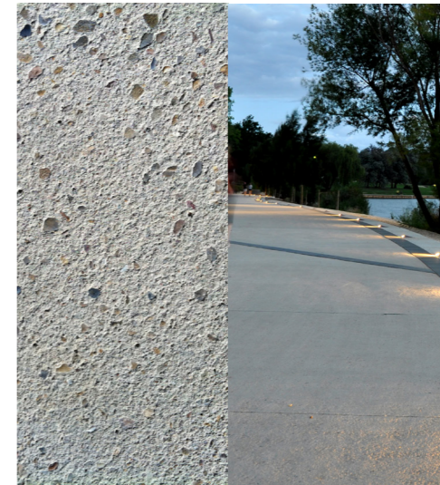
INSITU CONCRETE NON-SLIP FINISH LIGHTLY EXPOSED
