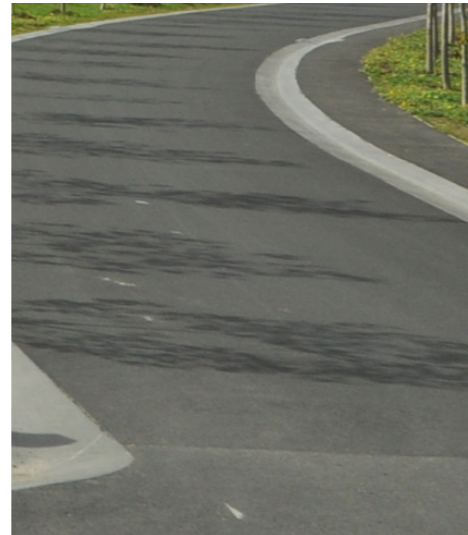
HOTMIX BLACK ASPHALTIC CONCRETE WIDE CONCRETE EDGING
