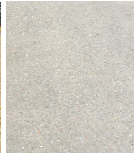
CONCRETE NON-SLIP BURNISHED FINISH
