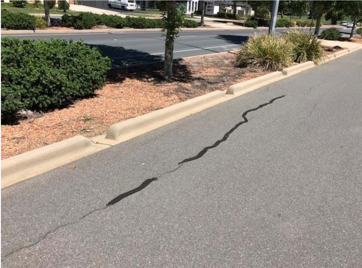
Figure 14. Example of an Open Kerb
