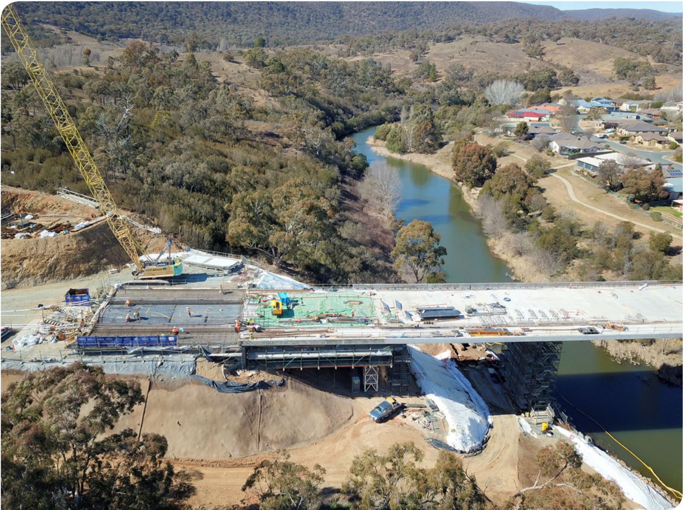
Work on launching bridge segments over the Queanbeyan River continues
