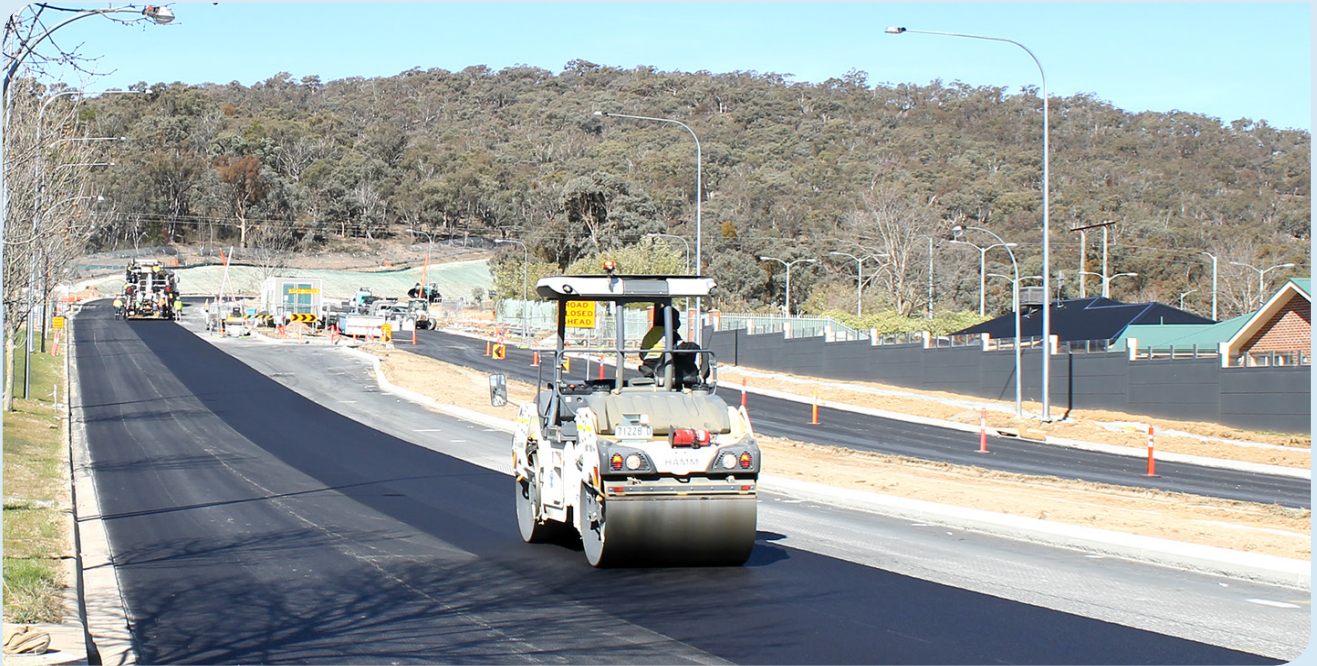
Work progressing on upgrade of existing Ellerton Drive
