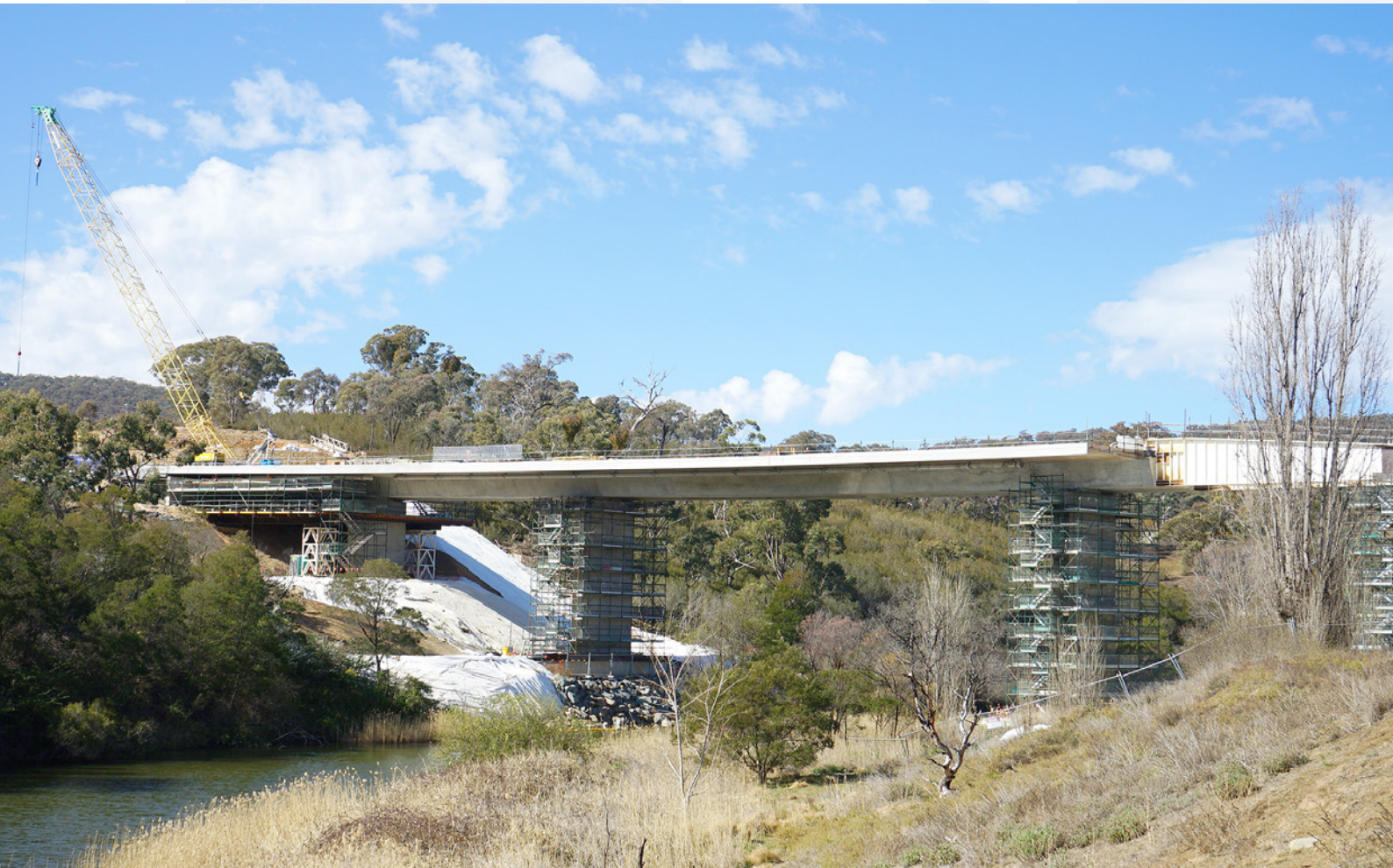
Bridge construction progressing over the Queanbeyan River, looking east
