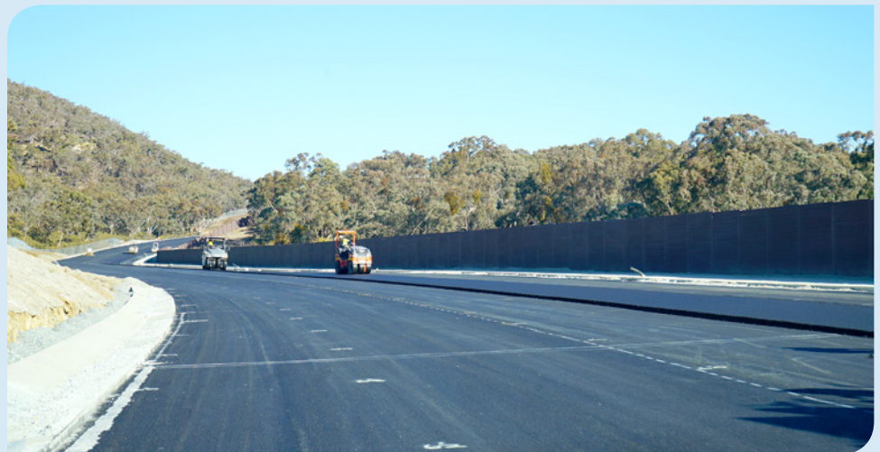
Pavement work underway on the northern side of the project
