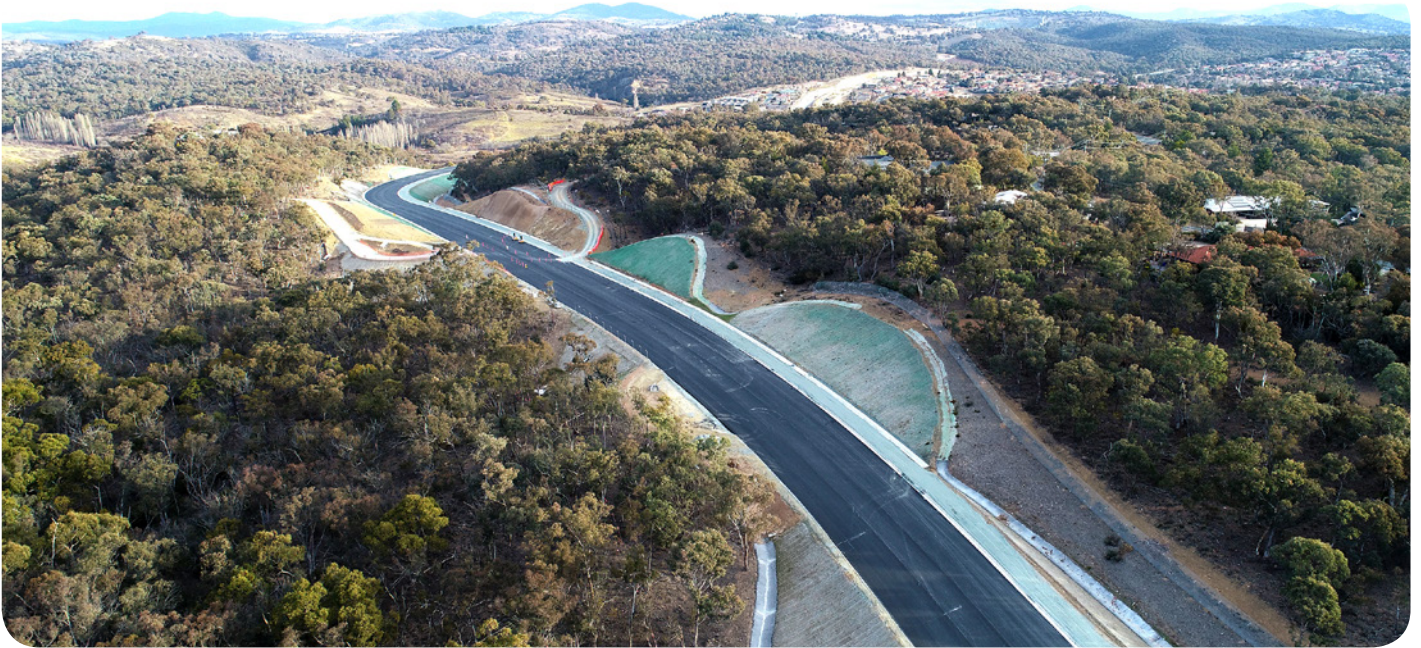
Project progress near Greenleigh, looking south
