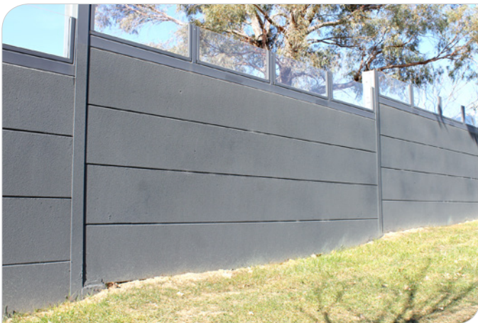
Completed noise wall on existing Ellerton Drive
