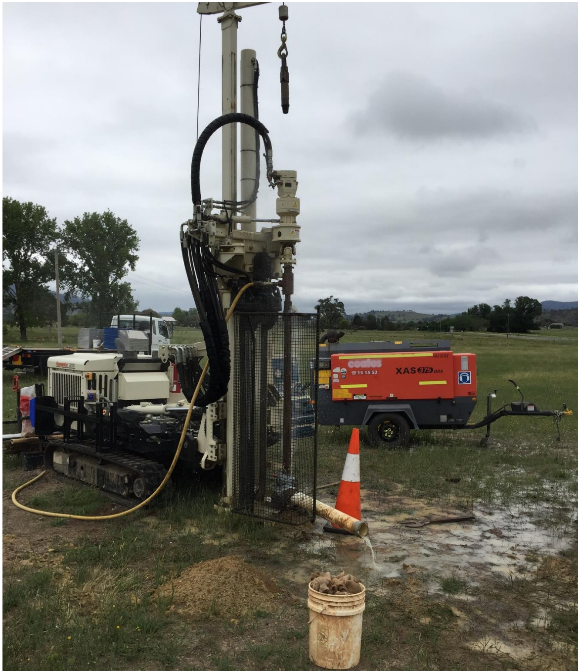
Figure 5 - Groundwater encountered during drilling for MW02B, using an air hammer attachment.
