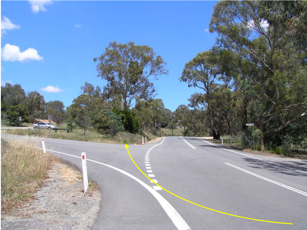
Plate 5. Old Cooma Road veers right (westwards) south of the Tempe Crescent intersection, located to the left (east). Stage 1 would be aligned between the two roads, as shown in the photograph.
