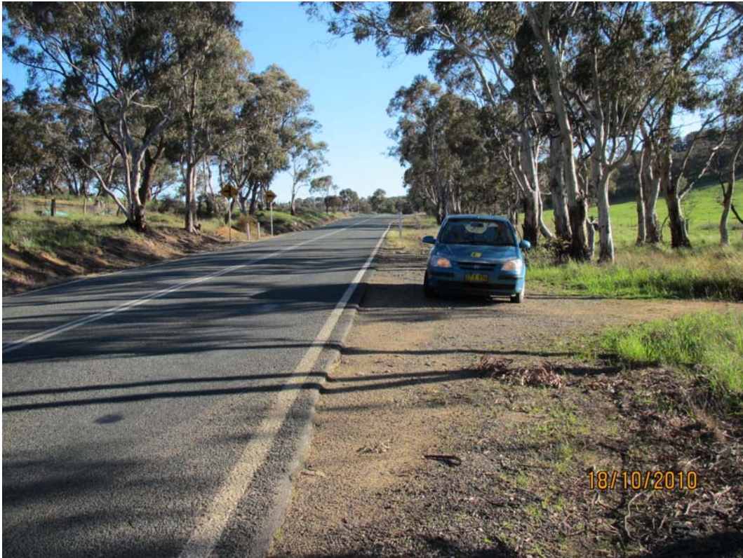
Plate 17. The photograph shows the southernmost section of the proposed duplication, with the turnoff to Googong Road in the background and the Googong Travelling Stock Reserve on the right.
