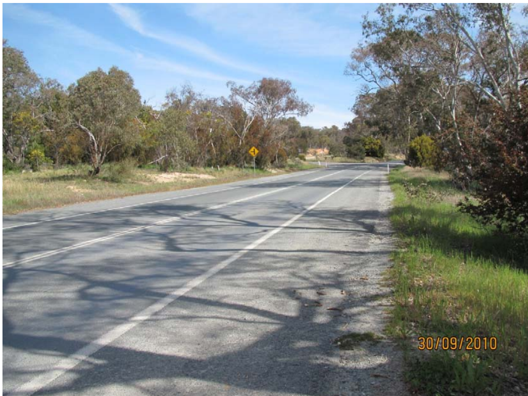
Plate 4. Old Cooma Road continues to the end of this section, where the road starts to bend westwards and uphill towards the Cooma Road Quarry, after the intersection with Tempe Crescent.
