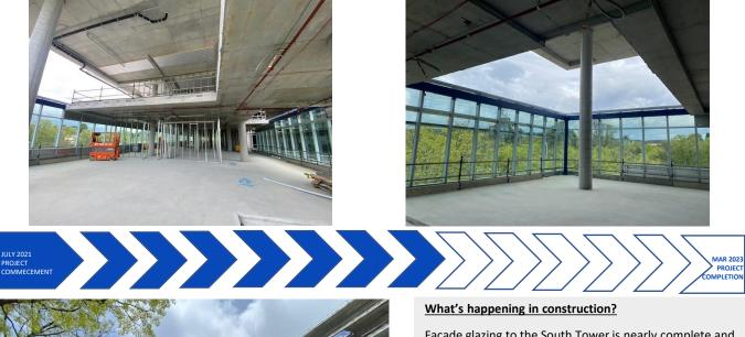
Façade glazing to the South Tower is nearly complete and works to Level 3 of the North Tower will start soon. Framing inside the building is well underway with Ground Floor to Level 2 frames nearing completion. This will allow for the service trades to finish rough-in works and start internal linings.
